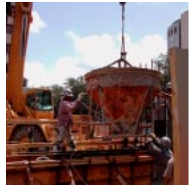
Workmen pour concrete into molds for positioning beamwork over Harris Gully.
