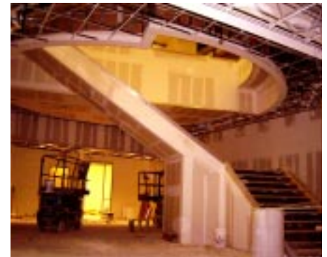
The grand staircase work progresses.
