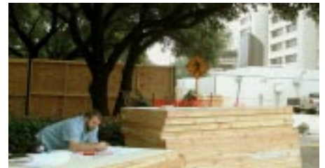
Marvin Allison, electrical foreman, Design Electric, works on berm project plans on the Fannin side of the Medical School.
